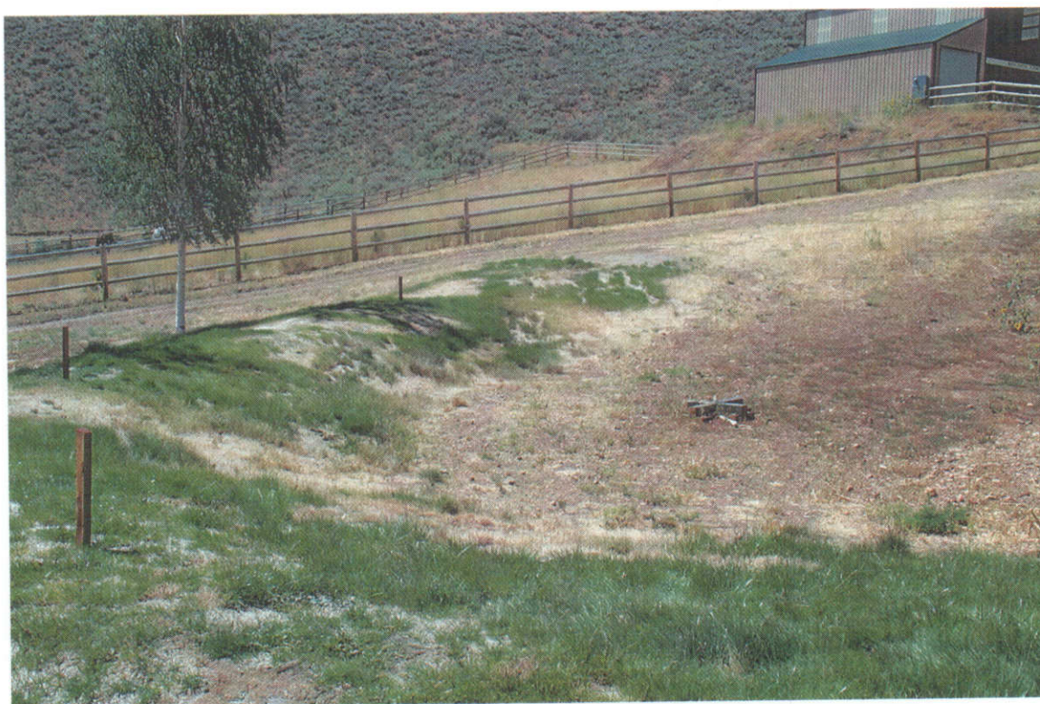
Existing Dam & Pond Area Looking SW By J E Stanton 8-13-2002
