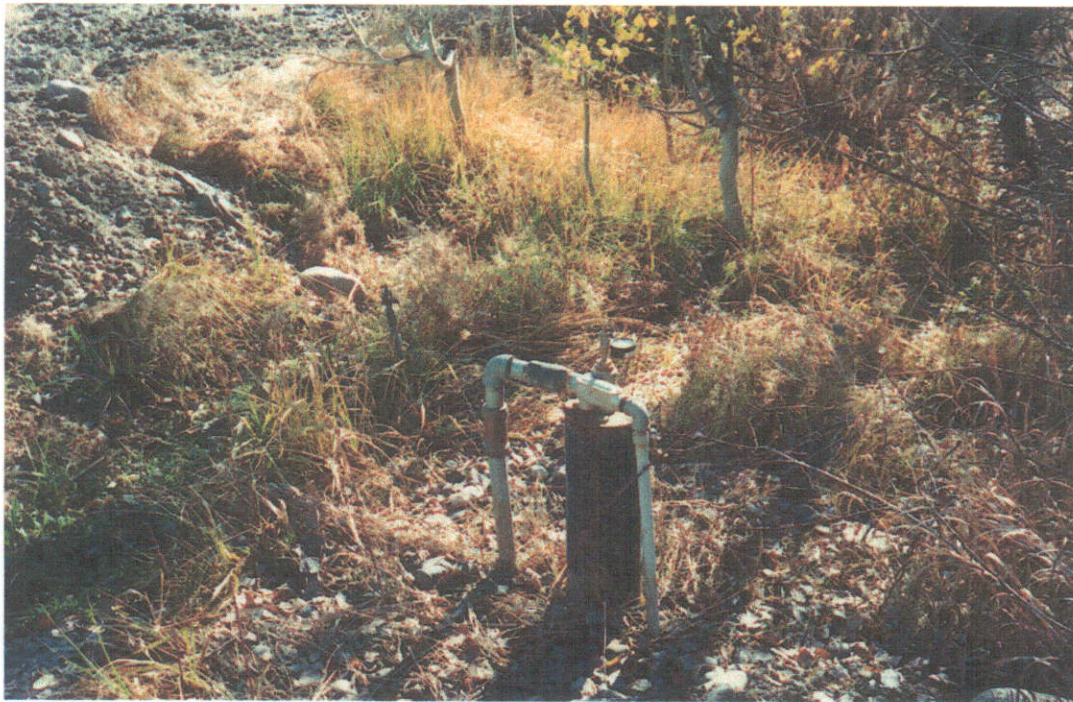
6" Dia Irrigation Well
