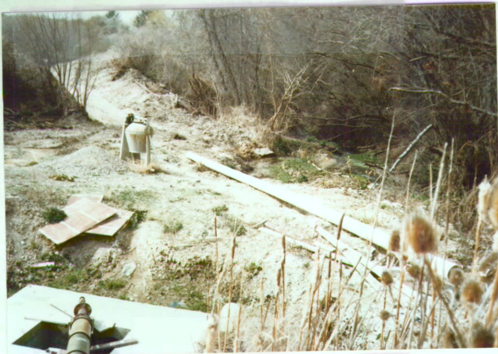
Menchaca Power Plant
