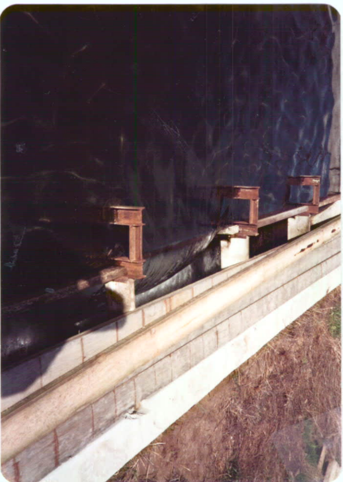
CHANNEL CONVEYING THE SPRING WATER TO THE RACEWAYS.
