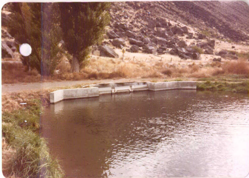
Inlet of Upper Pond
