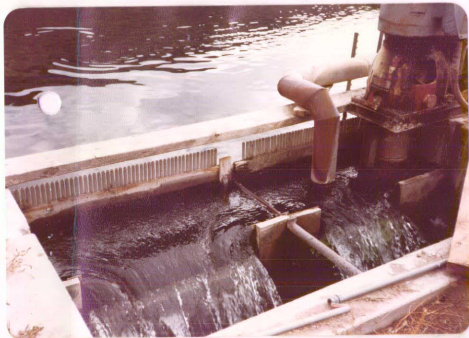
lower weir- outlet of upper pond
