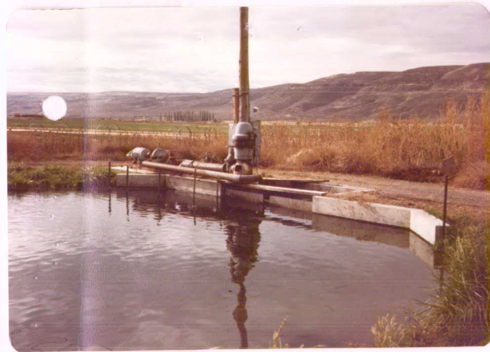
outlet of upper pond
