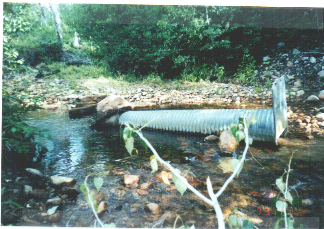
Diversion Structure In Soldier Cr. (Looking NE)
