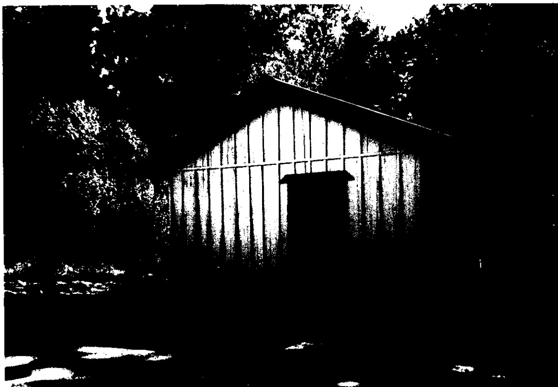
Pump House On East Side of Soldier Cr. Road
