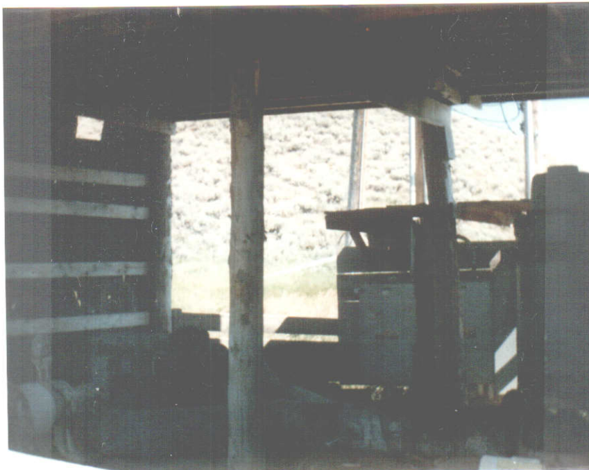
Point of diversion is located on right side. Boosters located in bottom left corner and left of middle.
