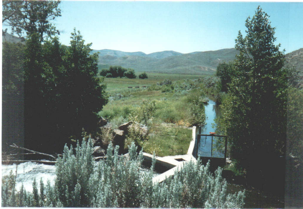
Upper diversion From West Canal
