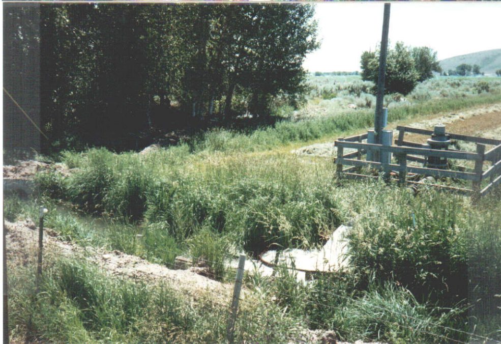
Diversion Works Discharge into Lower Ditch
