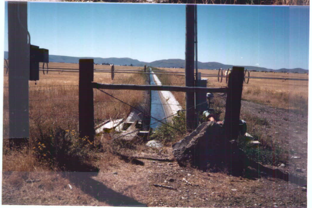
Ditch running south from pond at Well #2
