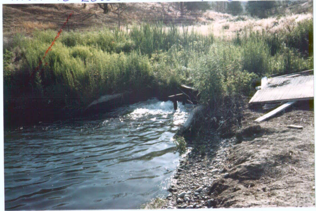
inlet to Lower Ponds Nth SIDE
