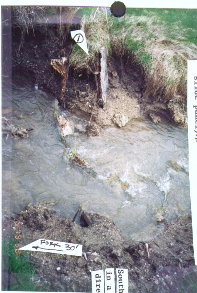
THIS IS THE OLD DIVERSION SYSTEM, (PUTTED AWAY BY LIMESTONE PER SCOTT CURTIS)
