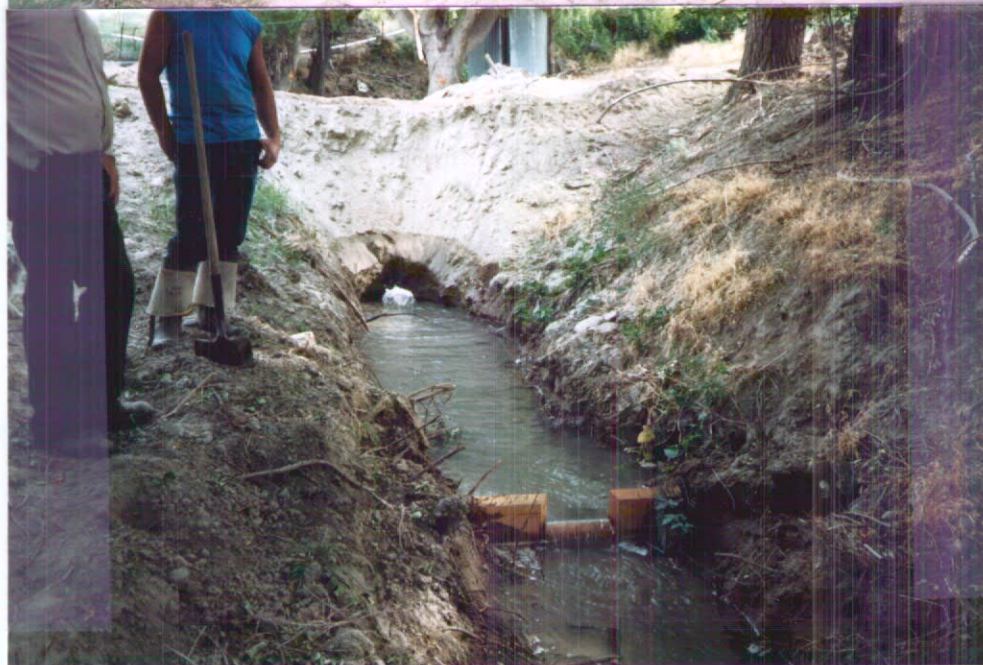
1' contracted rectangular weir mess. total output from spring. when pump turned on pump easily adjusted to consume total flow. During exam pump started and outflow ceased to flow.
