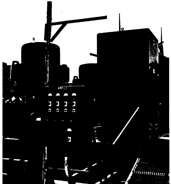
Four 2000 H.P. 2300 V. Panels and One 2000 Amp. Air Breaker Panel
