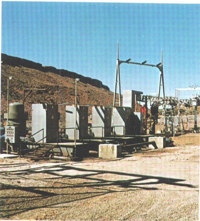
Four 2000 H.P. 2300 V. Panels and One 2000 Amp. Air Breaker Panel
