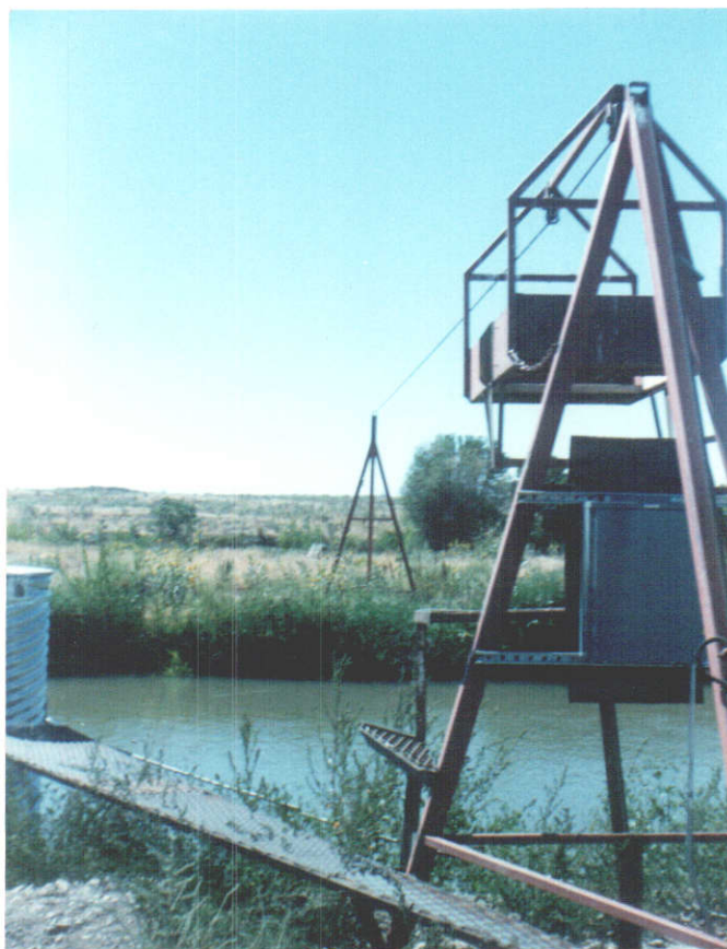
GAGING STATION ON POWER CANAL
