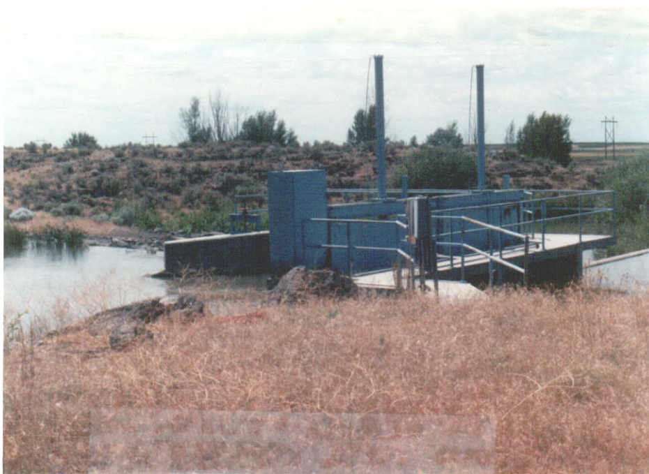
Control gates. Forebay on left. Feeder canal on right.
