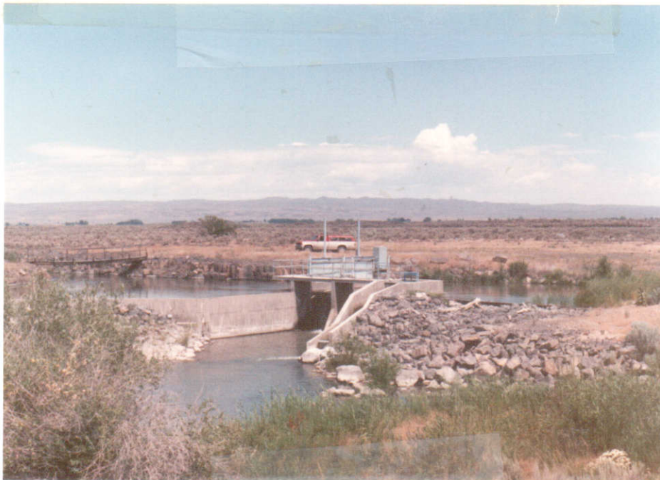
Looking upstream at the gates, spillways, downstream and measuring bridge on far left
