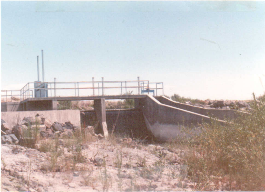
Looking upstream at feeder canal retaining wall on left, gate controls upper left, spill gates in center and low flow control in sluiceway on right
