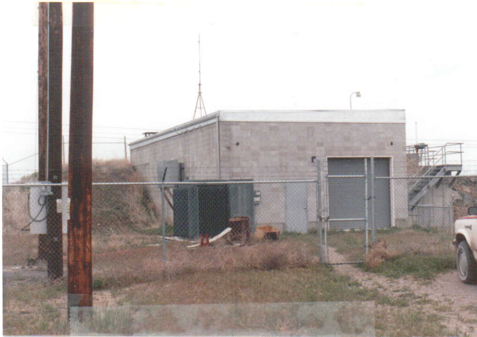
Powerhouse. Tailrace is in excavated canyon on right. Permit 37-7943
