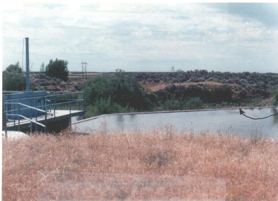
Concrete wall and spillway at head of feeder canal Permit 37-7943
