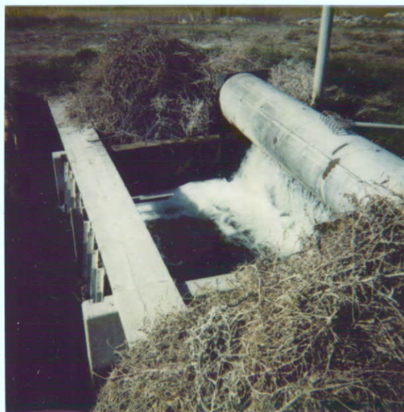
Div. Works + Canal to Penstock
