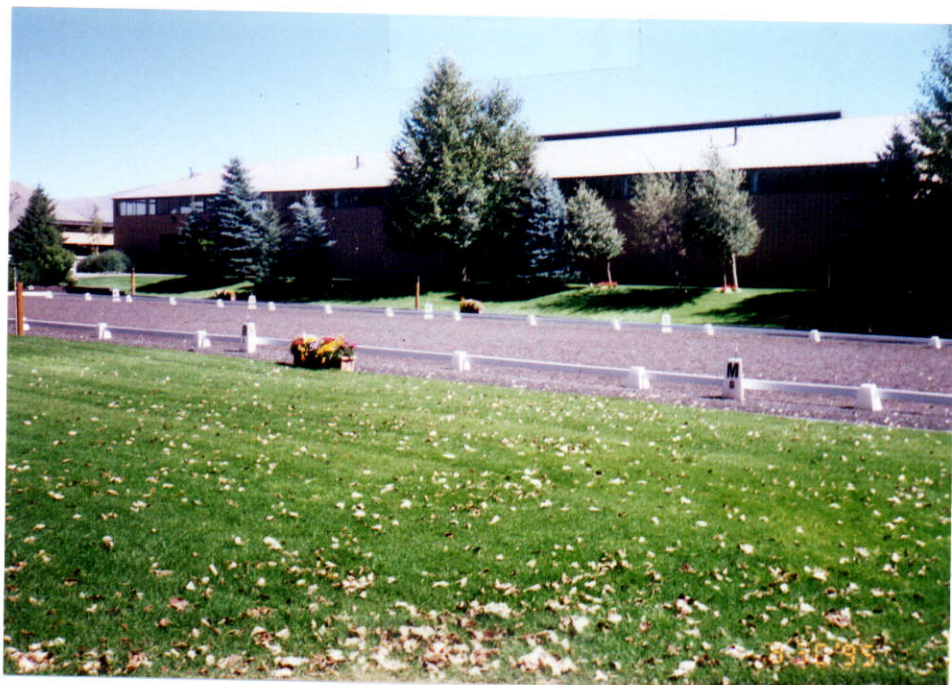
P.O.U. IRRIGATION + Commercial SHOWING INSIDE ARENA (BACKGROUND) OUTSIDE + ARENA (FOREGROUND)
