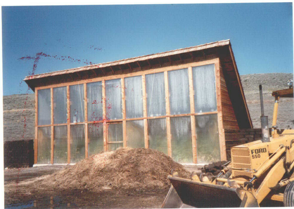
Solar Heated Green House. Looking North
