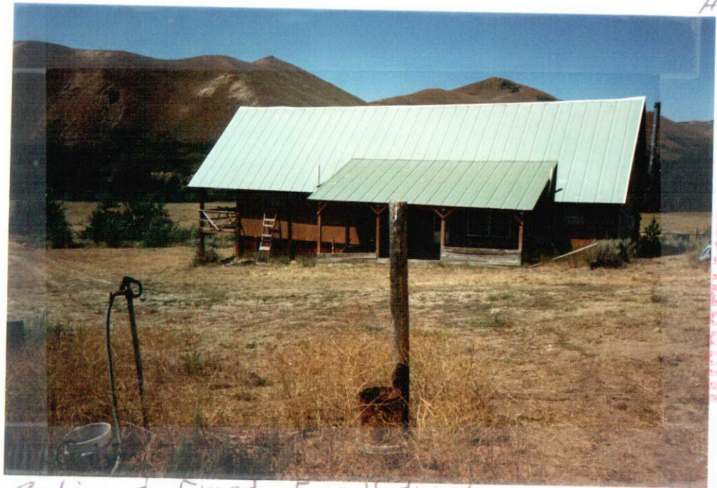
Cabin & Frost Free Hydrant.
