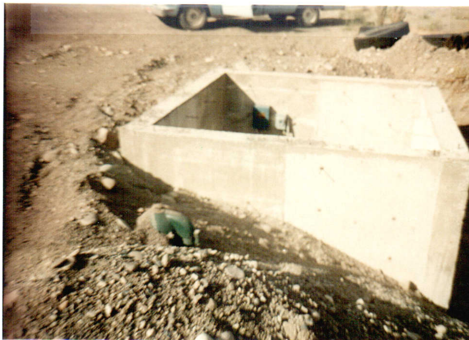
P.O. Looking west
