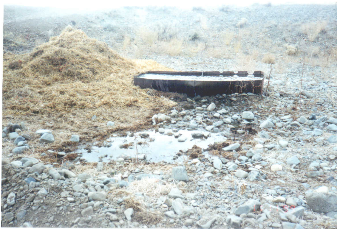
Stock Trough Looking South
