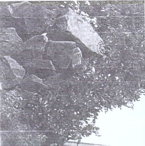
Back of pump house; outlet for overflow from cistern
