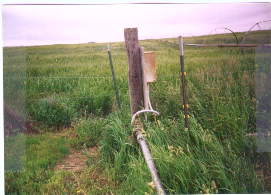
P/D - well cap IMMEDIATELY TO THE LEFT OF THE RISER.
