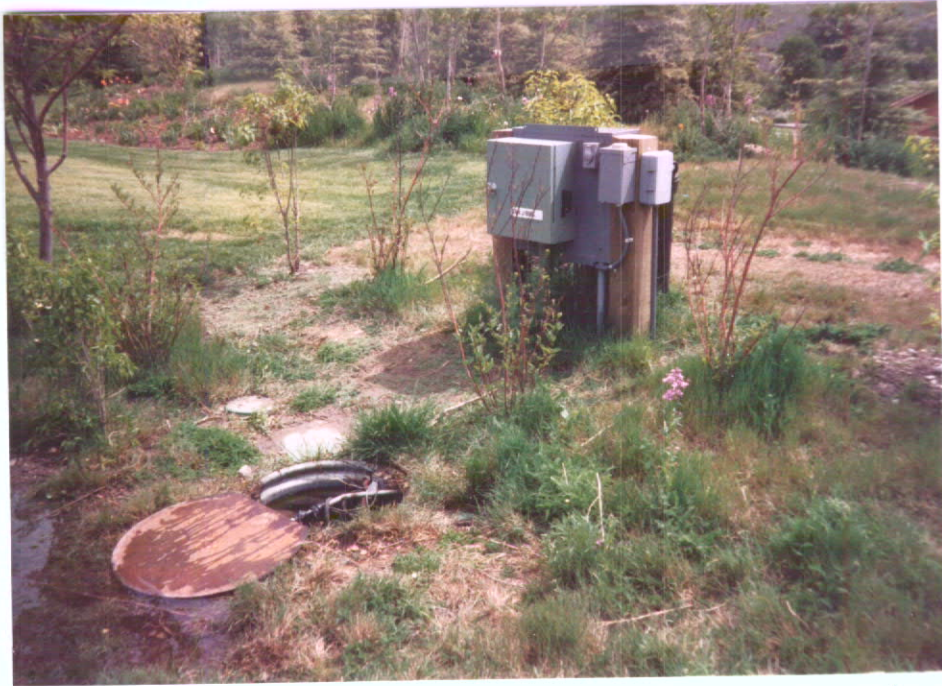
pond pumping set up & sprinkler box
