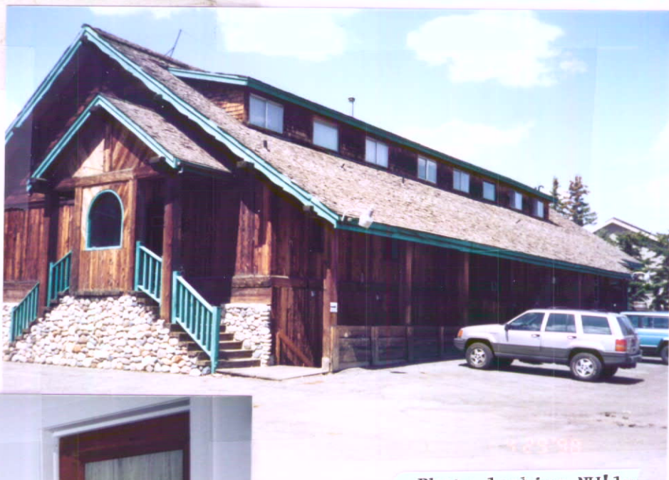
Photo looking NW'ly south end of bldg.
