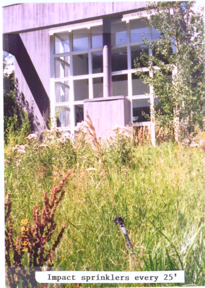
Impact Sprinklers at frontage of the Hyndman View Drive.
