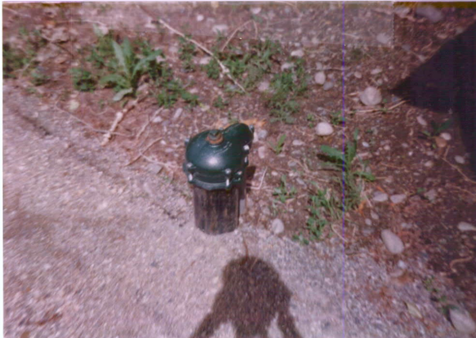
P/D #2 Backup well
