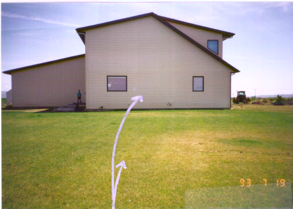
P/U This photo is taken from the row of trees looking west. The lawn is included in the irrigation component of permit.
