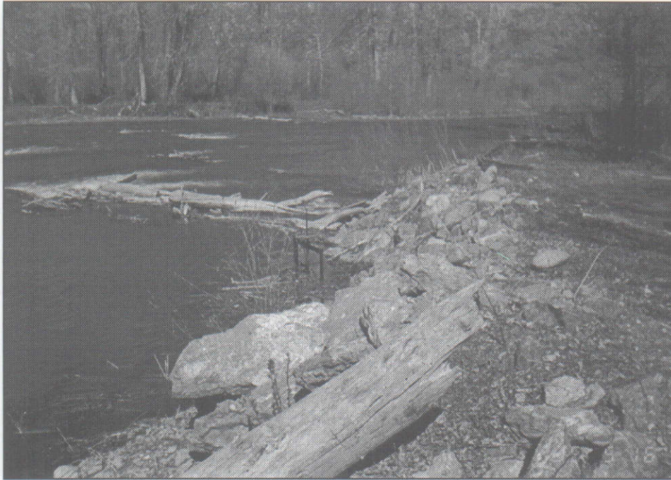
Figure 1. Comstock Ditch diversion from Big Wood River.
