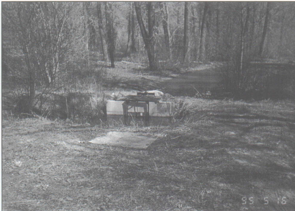
Figure 2. Comstock Ditch submerged orifice and River's Edge pond No. 1.
