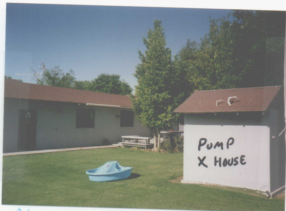
P/U - HOUSE , ALSO P/O LOCATION
