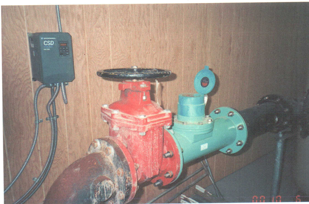
6" Water Specialties Meter - Serial #9317186 - Model ML-04 - Calibrated 5/6/97
