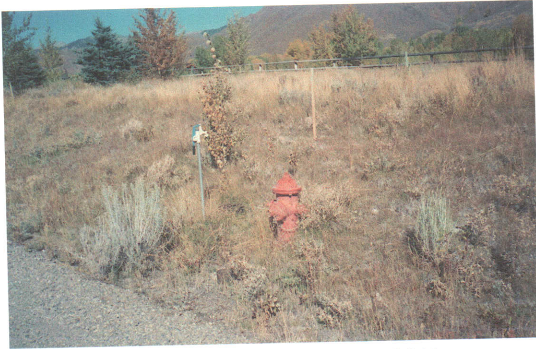
Fire hydrant & Yard Hydrant - Total = 2 within subdivision
