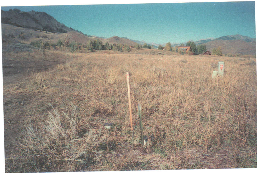
Domestic stub out location - marked with steel fence post
