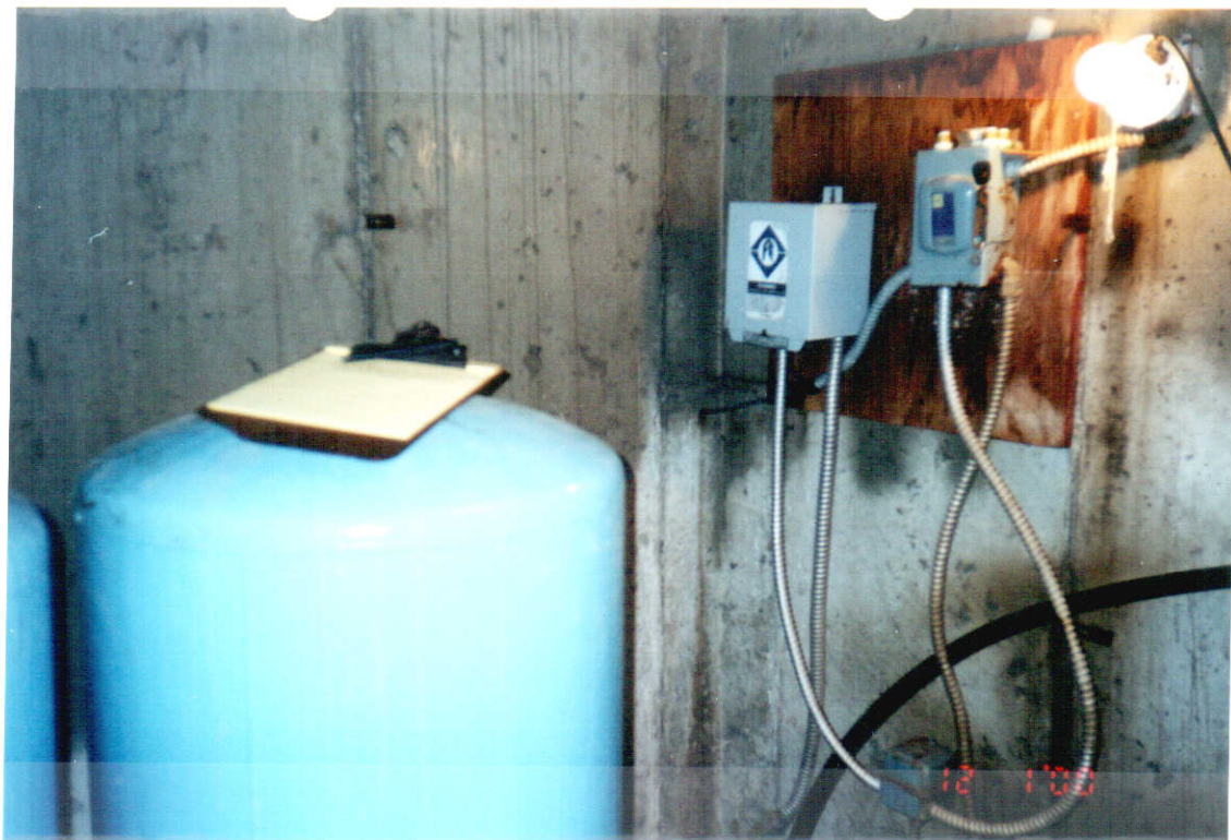
Inside of Well House
