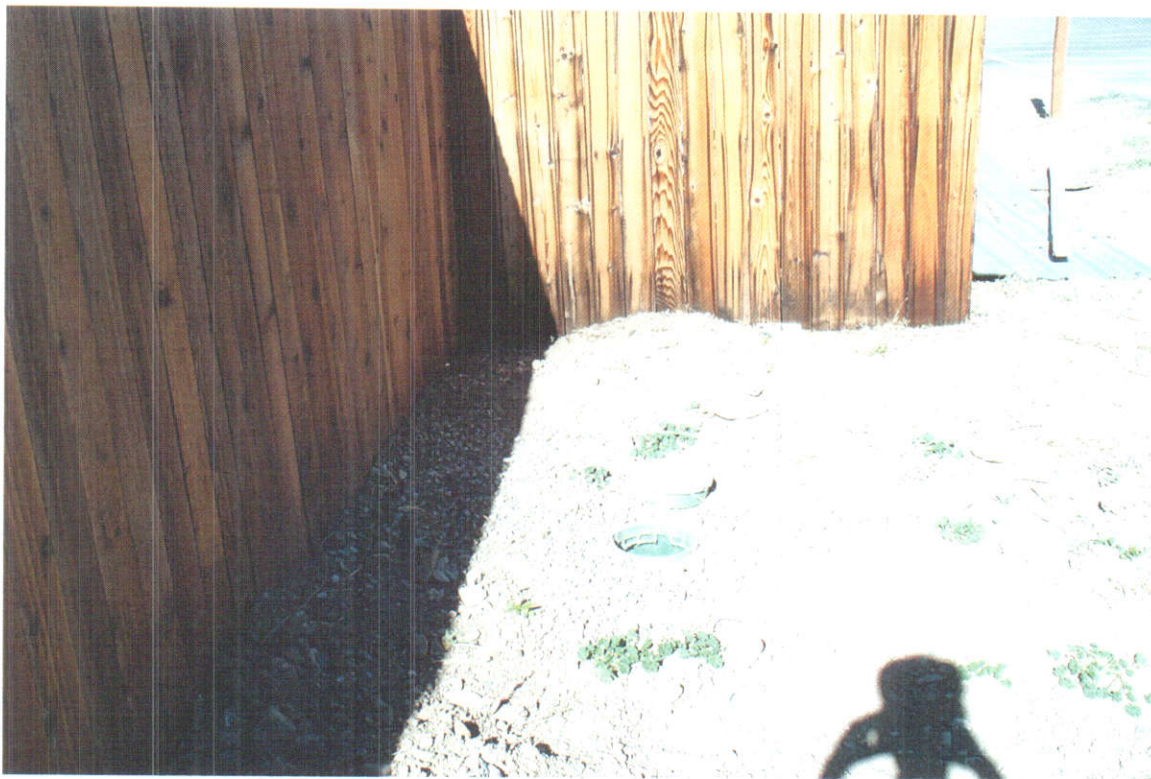
Location of Flow Sensor East of Well Enclosure By J E Stanton 10-9-2002 Permit 37-8821
