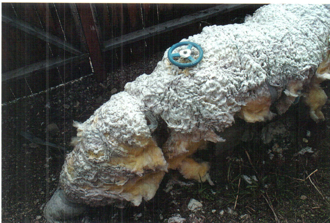
Mainline Going Underground East of Well By J E Stanton 5-2-02
