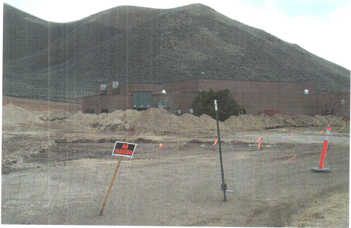
Area At North End of High School Torn Up For Construction Of New High School. By J E Stanton 5-2-02 37-8821
