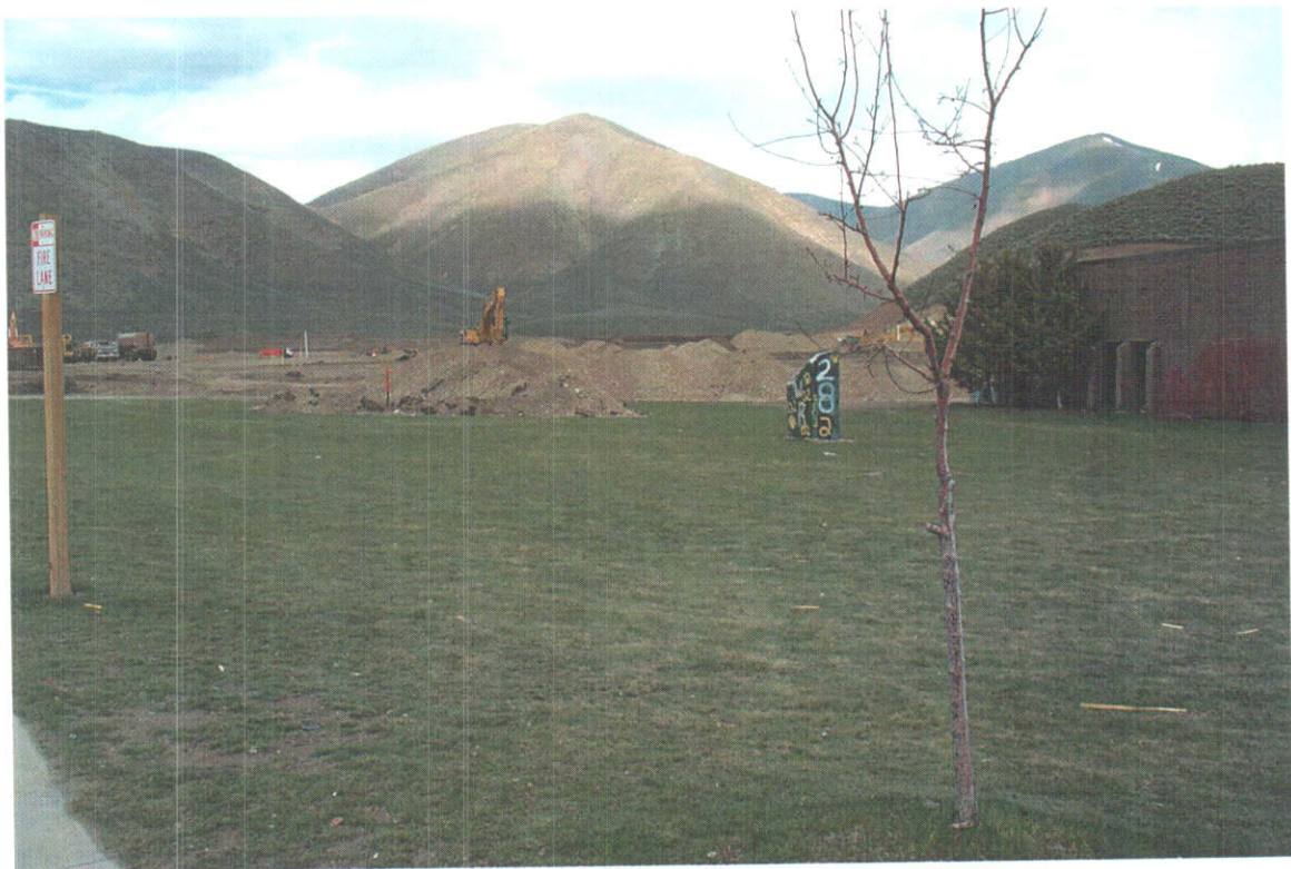
Lawn On West Side of High School Looking North From Main Entrance (Some Lawn Already Torn Up Due To Construction Of New Building) By J E Stanton 5-2-2002
