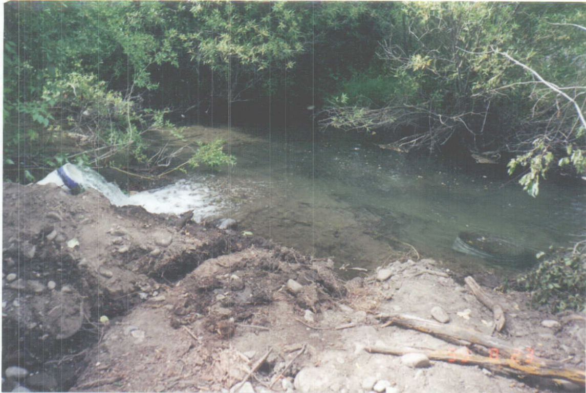
PICTURE SHOWS INLET CMP PIPE & OUTLET SPILLWAY PVC PIPE. DISTANCE FROM INLET TO OUTLET IS APPROX 15 FEET.
