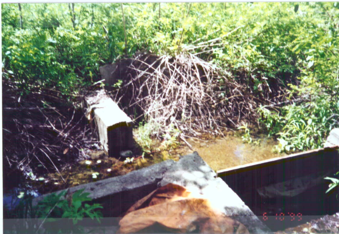
Splitter Box On Wrencher Ditch
