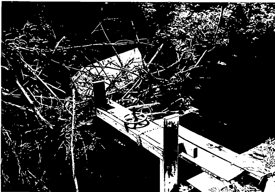
Headgate on Agway Broadford Slough
