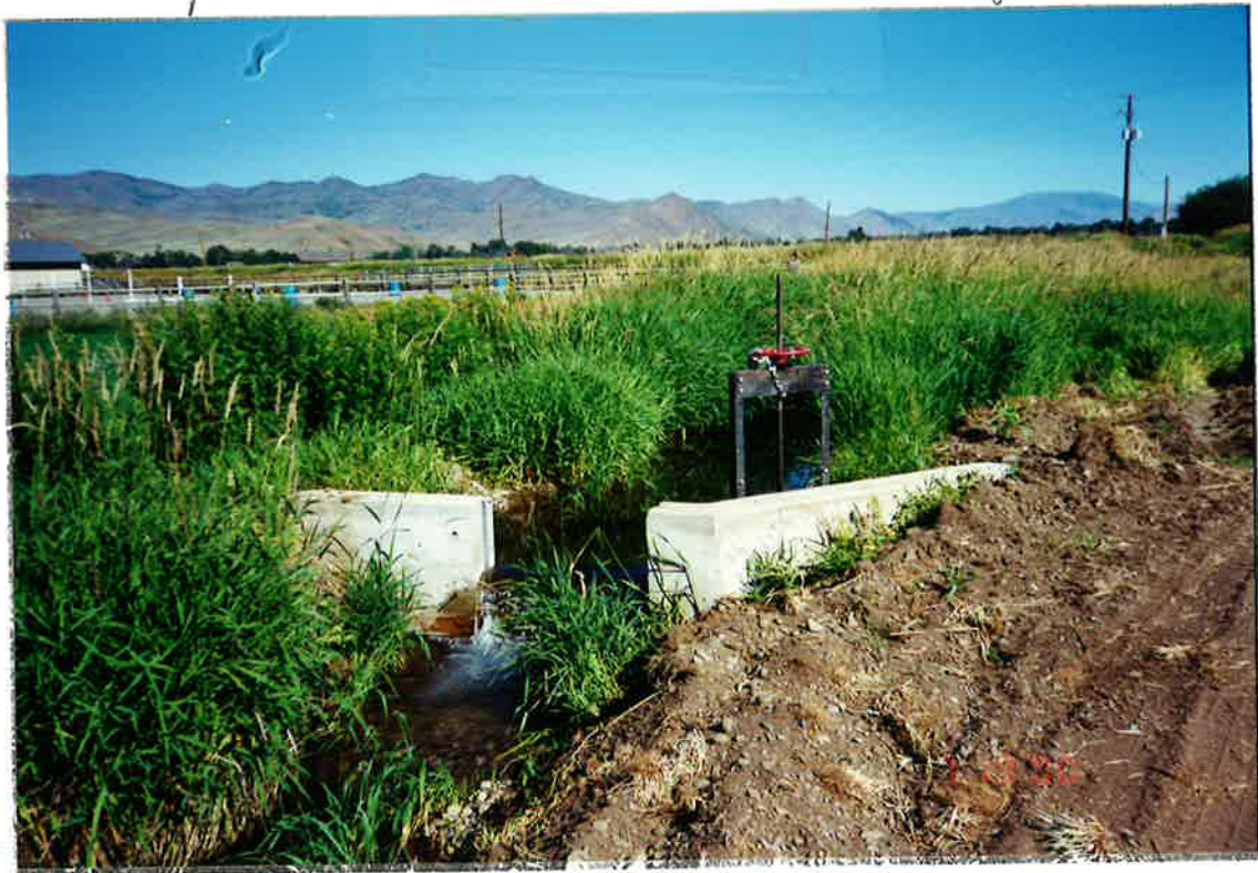
Headgate In Ditch To Bloomfield Pond (Looking N)
