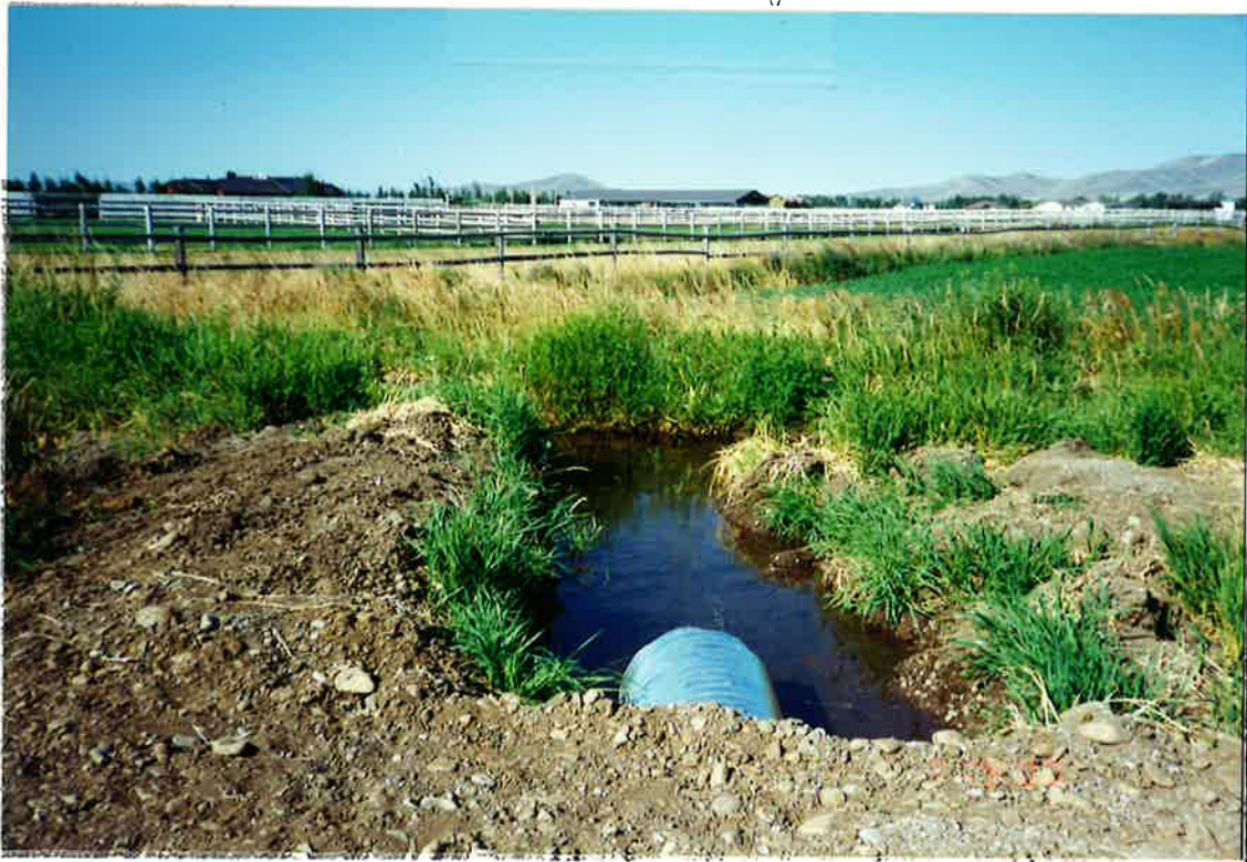
Point Where Pond Outflow Re-Enters Irrigation Ditch
