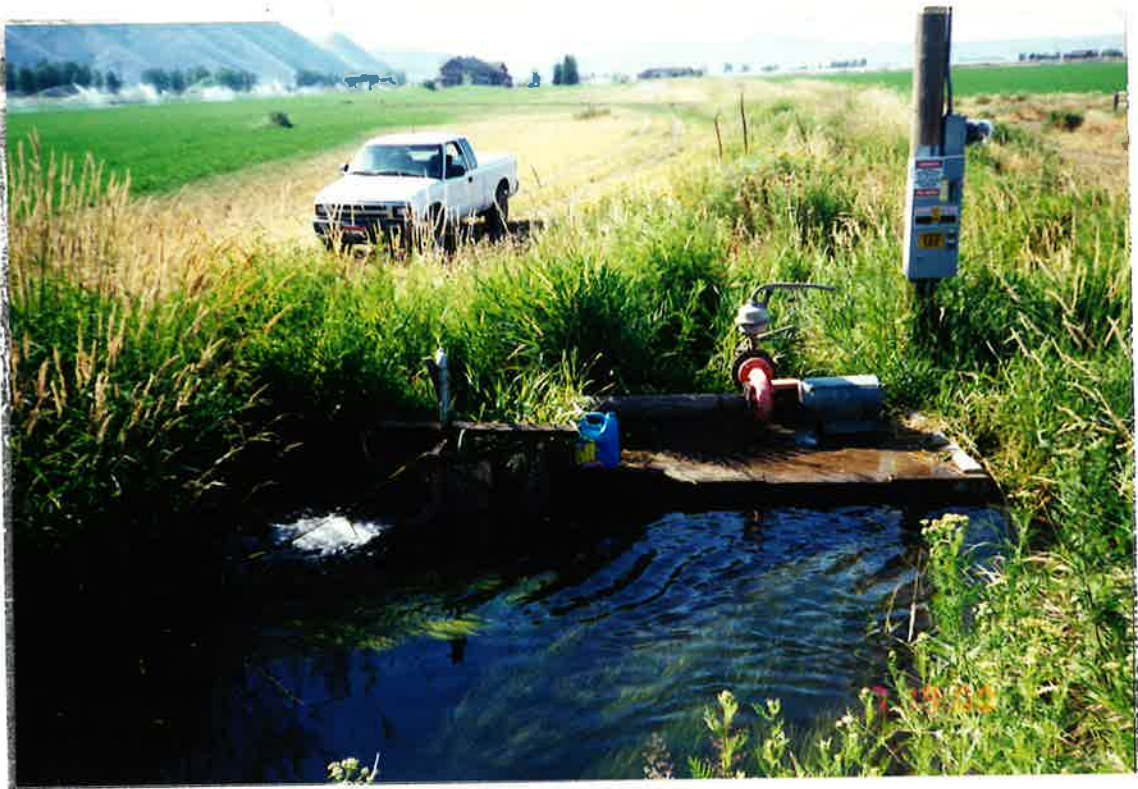
Pump Diversion N of Bloomfield Place (Looking South)
