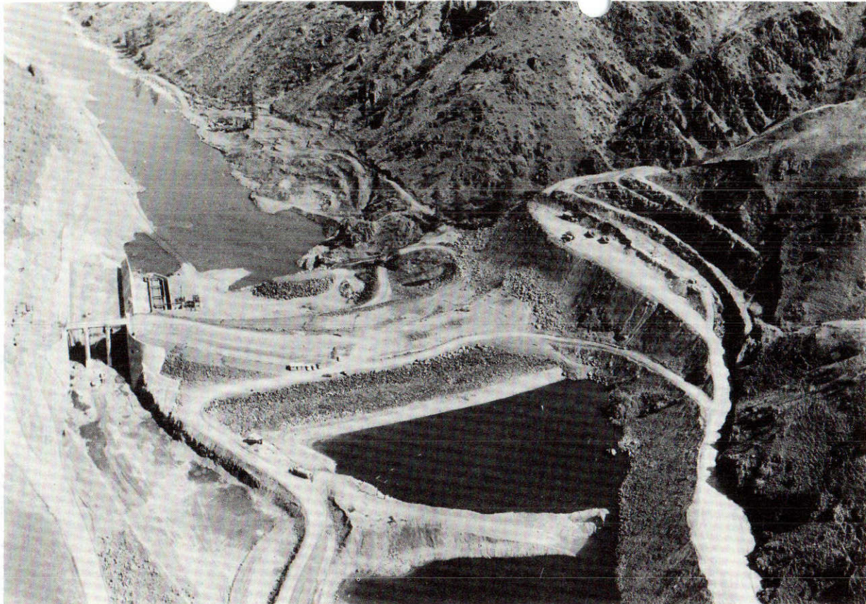
AERIAL VIEW shows broad spread of work being performed in the big Oxbow project's dam area. Rockfill embankment is at center, within 50 feet of its final height. Concrete spillway and one of two upstream-migrant fish facilities are at left and excavation for fuse-plug spillway is under way on Idaho side of embankment at right.
