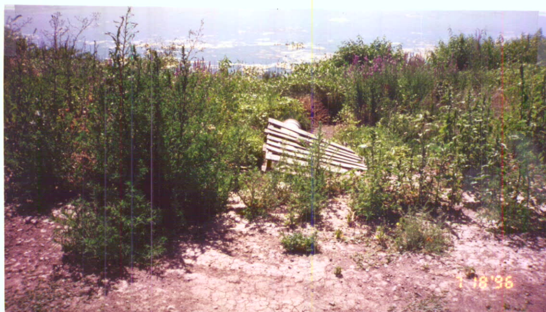
inlet pipe ft. res. to galloway pump
