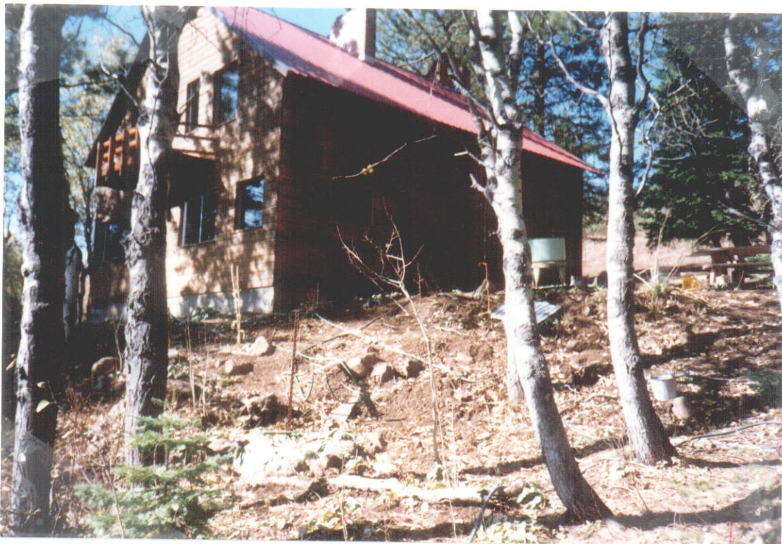
P.U. Cabin pipes & hoses are visible in lower center of photo Looking Northwest
