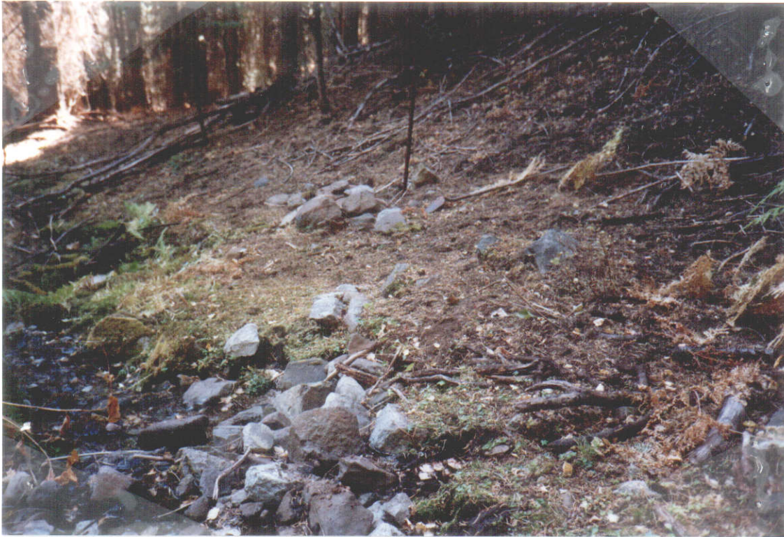
P.D. Creek is visible in lower left of photo. Stake (metal fence post) marks the corrugated pipes with screens (upper center of photo) Looking South-Southeast.
