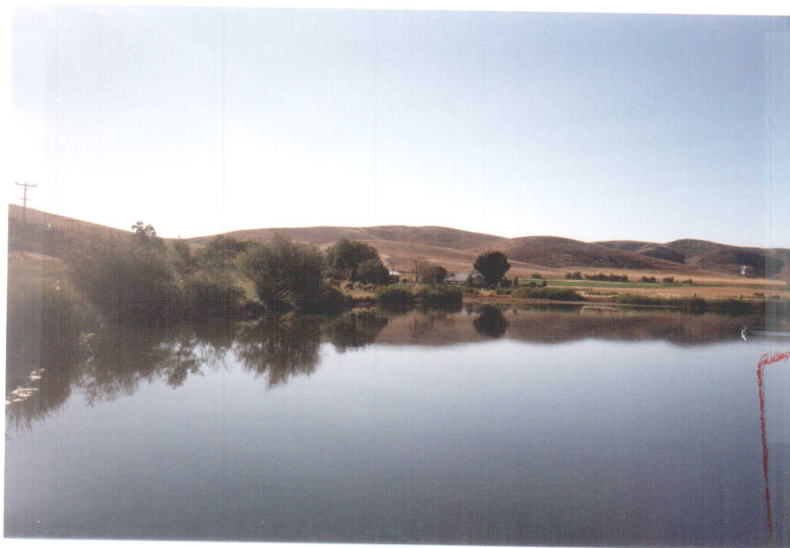
RESERVOIR + P. U. LOOKING EAST FROM DAM
