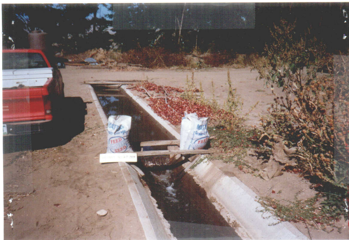
Weir Looking North (Pump had just been shut- off and the water level in the ditch was dropping.
