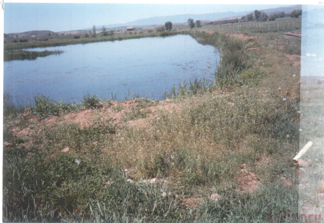
Pond #2 Pumps from this Pond. FEB 04 1993
