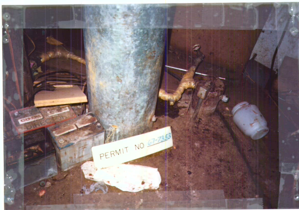
P.D. Facing Northwest inside the pumphouse/ shed.
