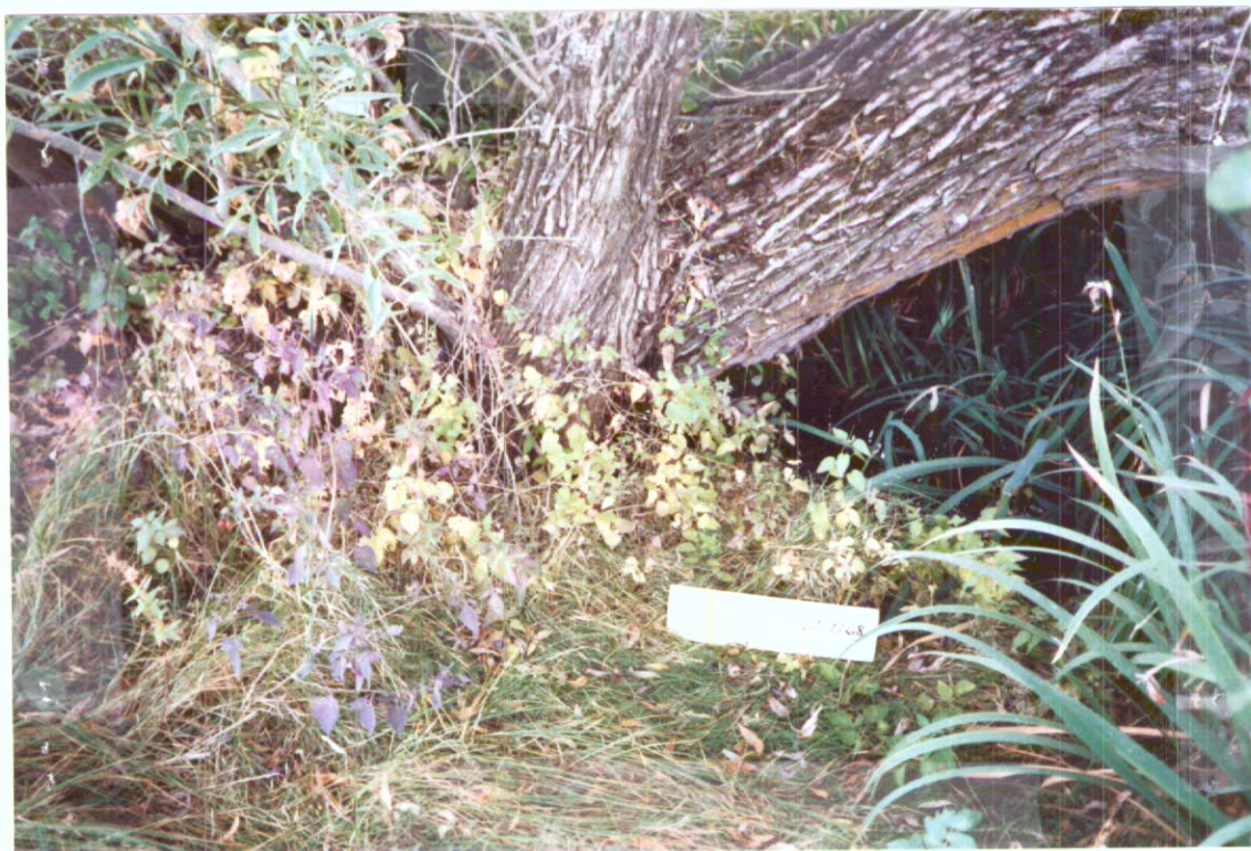
P.U. Looking Southeast A pool of water is below the tree limb.
