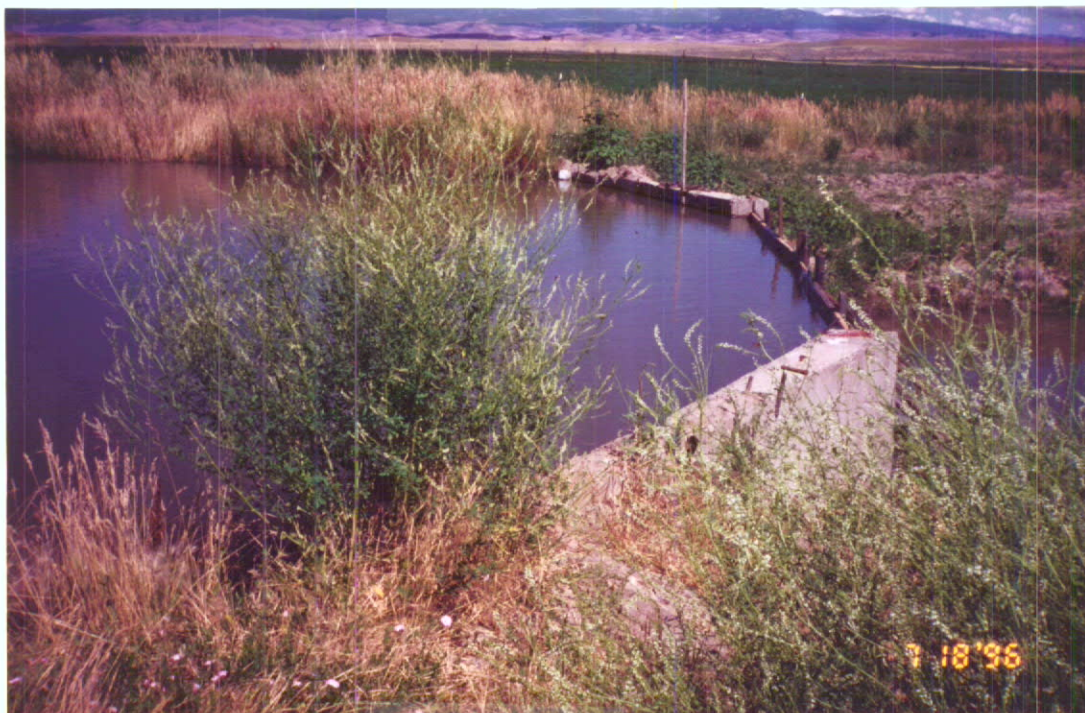
Check dam & pool in Hog Creek.
