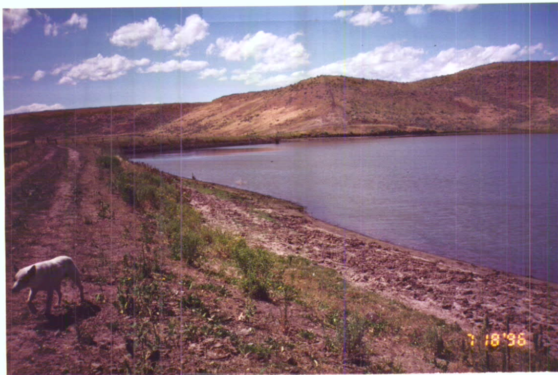
Dam SENE Sec 26 view to North
