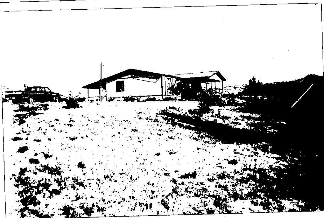
View of PHU looking South West. Water is PIPED INTO THE HOMES PRESSURE TANKS. THE LAWN IS IRRIGATED THROUGH RAUBERS FROM THE SPIGOTS.
