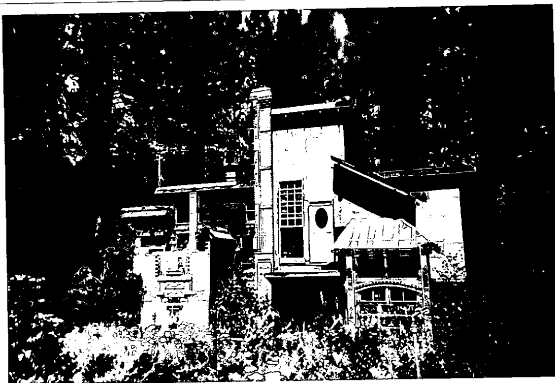
PHOTO THREE- View OF FRONT OF home.
