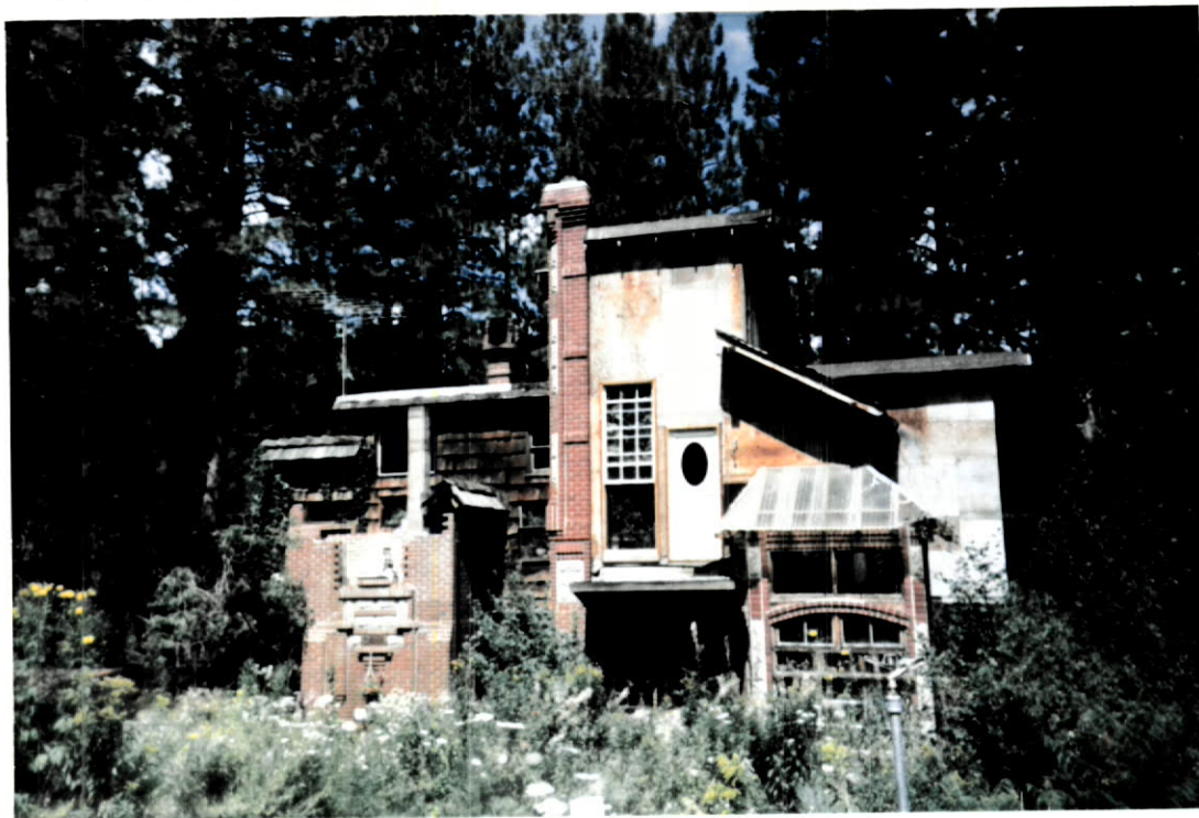
PHOTO THREE- View of front of home.
