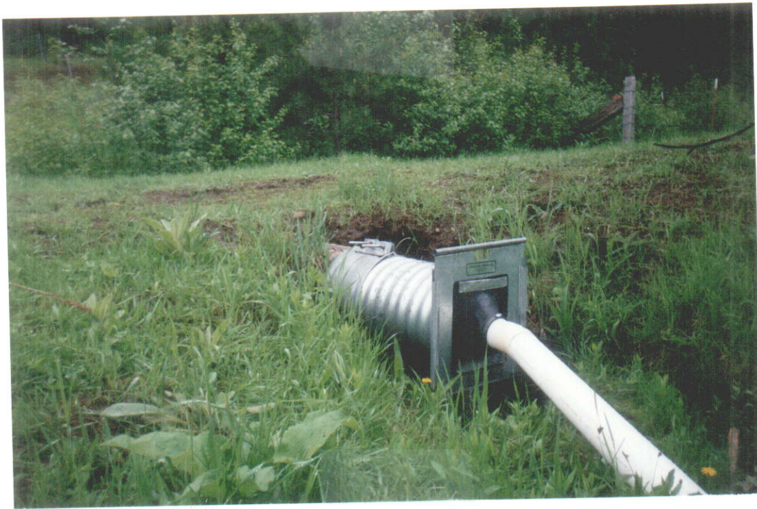
PHOTO ONE- Lockable Device (gate) attached to CMP under ROAD. TOTAL STREAM FLOW is diverted through 4" PVC to STOCK TROUGH.
