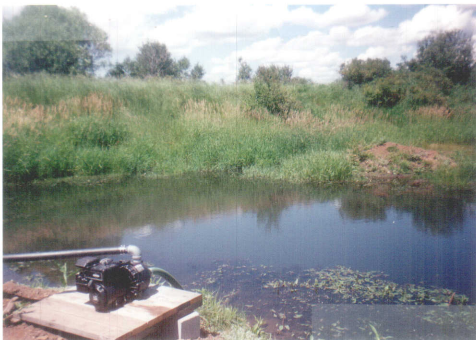
VIEW OF Pld. WATER IS PUMPED OUT OF THIS POND, UP A HILL (PLOT #2).
