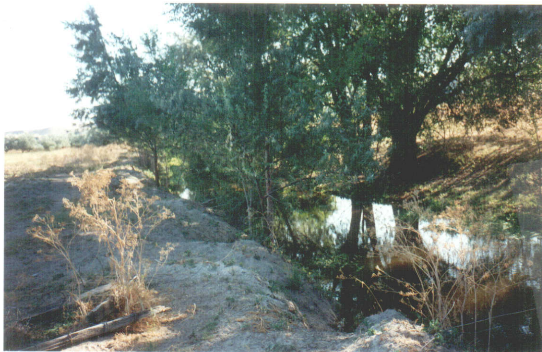
View of Drain AS IT CONTINUES ALONG THE P/U.
